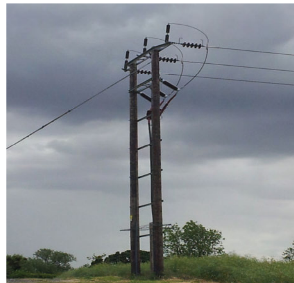
Appendix C- 2 Pictorial illustration of a H-pole that would be used to connect the underground cables on the overhead line circuit
