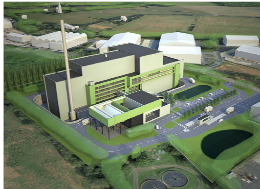
Image 4 - Aerial View from the North West
