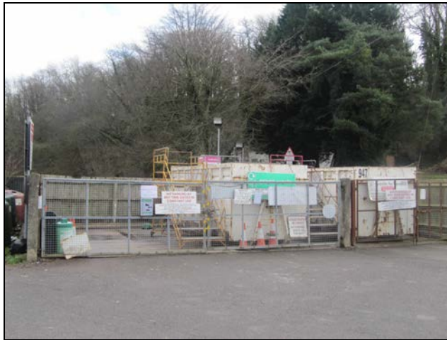
Plate TS1 – Existing Tenbury Wells Waste Drop Off Facility at Palmers Meadow
