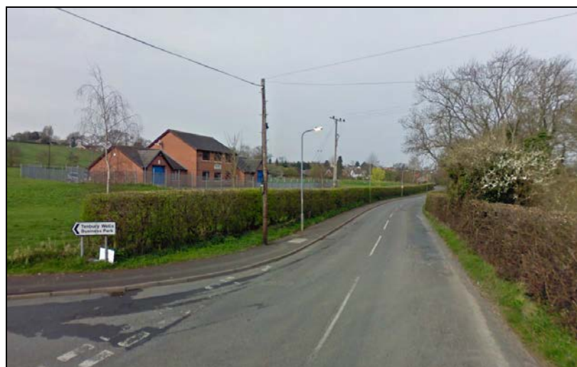
Plate TS6 - B4214 Bromyard Road West of Industrial Estate Access
